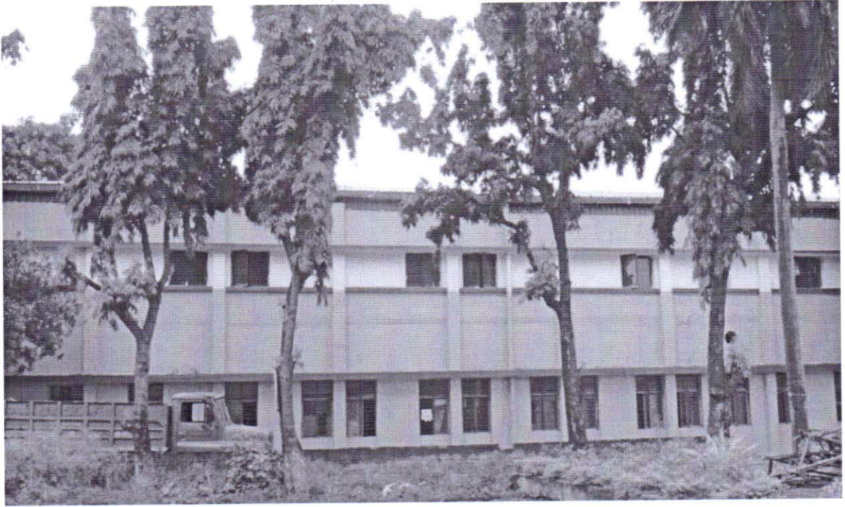
Rear view of the building
